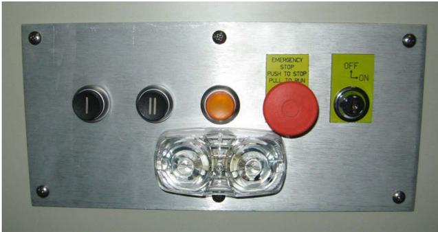
**Key switch:** Turn on to activate landing buttons (1 or 2)
